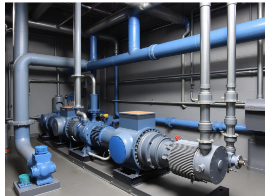
Pump room — MEP works
