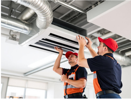
VRF installation — luxury villa
